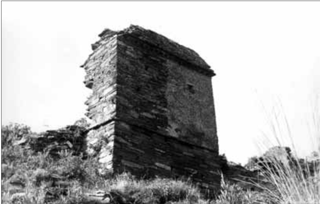
Fig. 504. Kanjar-Kote. Double vihara. N side with podium, substruction wall, cell and covering roof. (Taddei 1959; Neg. CS).
