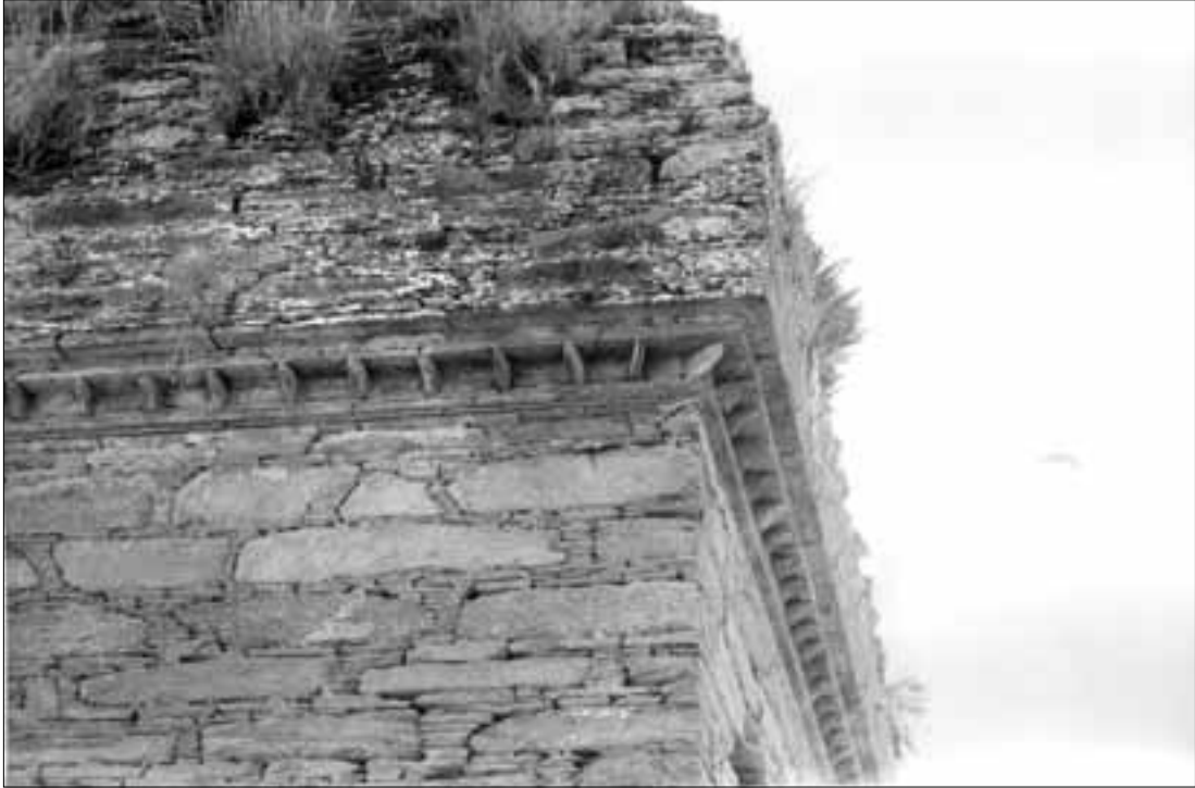
Fig. 471. Vihara of Gumbat. SE side; cornice of the lower roof covering. (Taddei 1959; Neg. CS).
