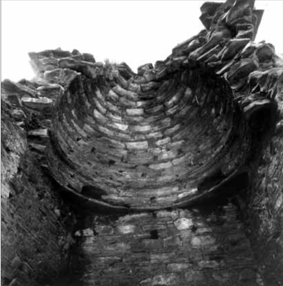
Fig. 446. Abbasahebchina, vihara F Inside of the aedicula (B); lower dome with springer on corner slabs and overlying band (F, G). (Kuwayama 1993).
