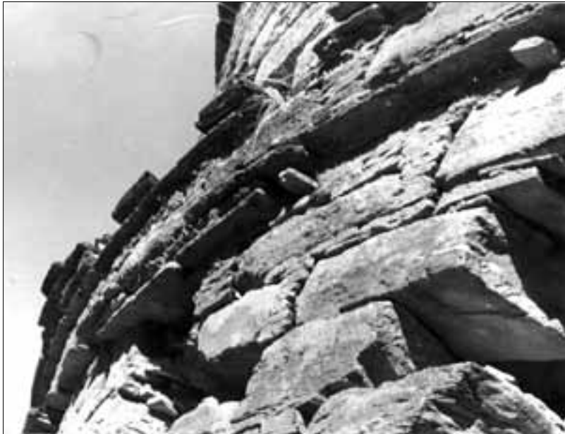
Fig. 393. Stupa of Top Dara (Haibatgram, Thana). SE side; 3 rd storey, detail showing a modillion of pilaster and cornice, profile view. (Nascari 1993; Neg. CS).
