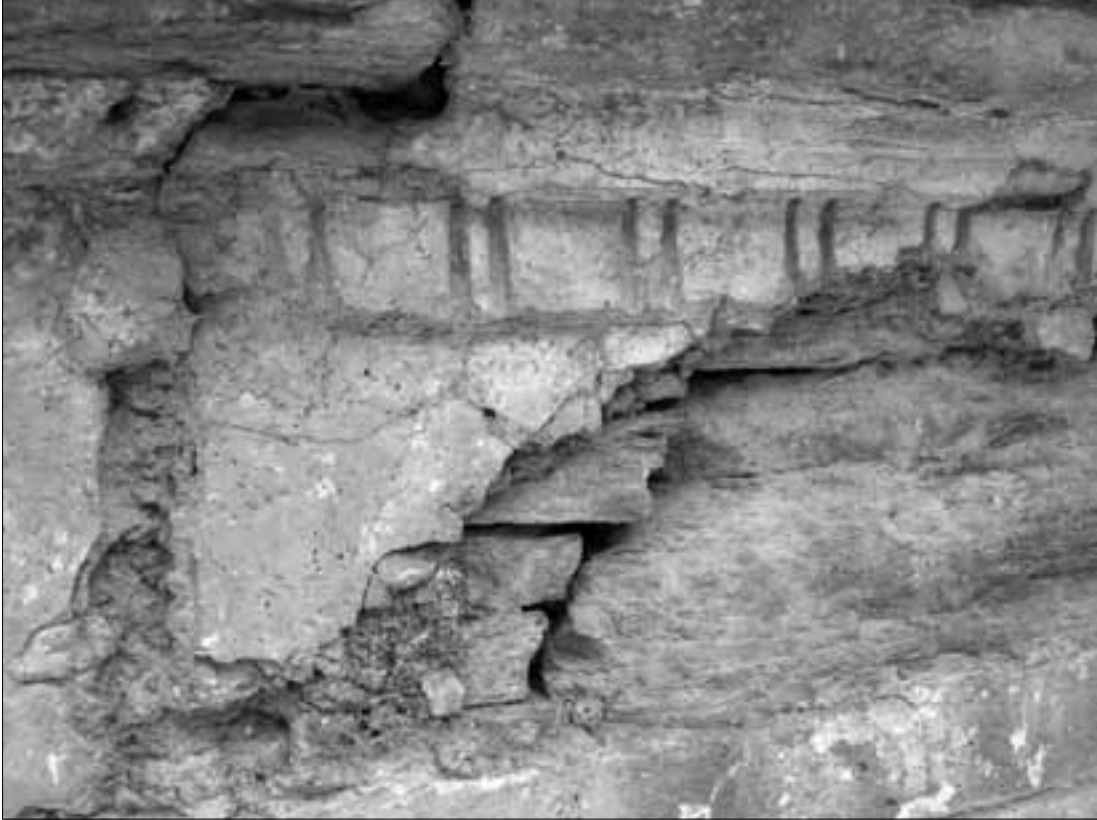
Fig. 303. Abbasahebchina. Stupa C. SE side, 3 rd storey; modillions of pilasters, stretch of architraved and bracketed cornice; plaster remains. (Spagnesi 2005).
