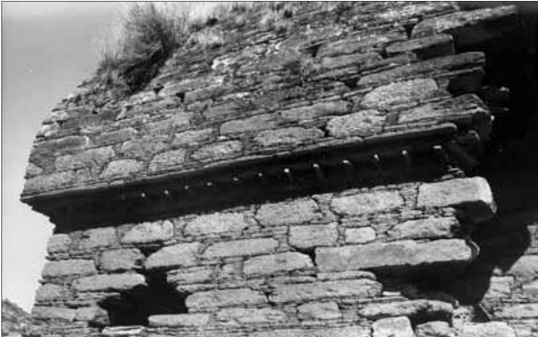
Fig. 465. Vihara of Gumbat. S side; cornice of the lower roof covering. (Taddei 1959; Neg. CS).
