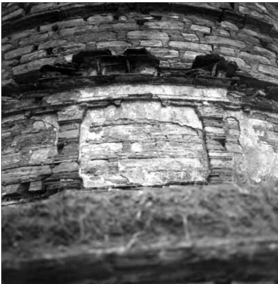
Fig. 241. Abbasahebchina. Stupa A. 3 rd storey (drum), 4 th storey (transition storey of the composite dome); with remains of plaster. (Kuwayama 1993).
