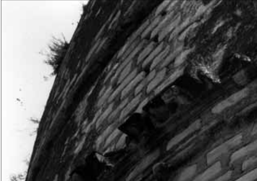
Fig. 146. Stupa of Shankardar. W side; 3 rd storey (drum) with pilasters, cornice with architrave and brackets; above the 4 th transition storey of the raised dome. (Sabelli 1993).
