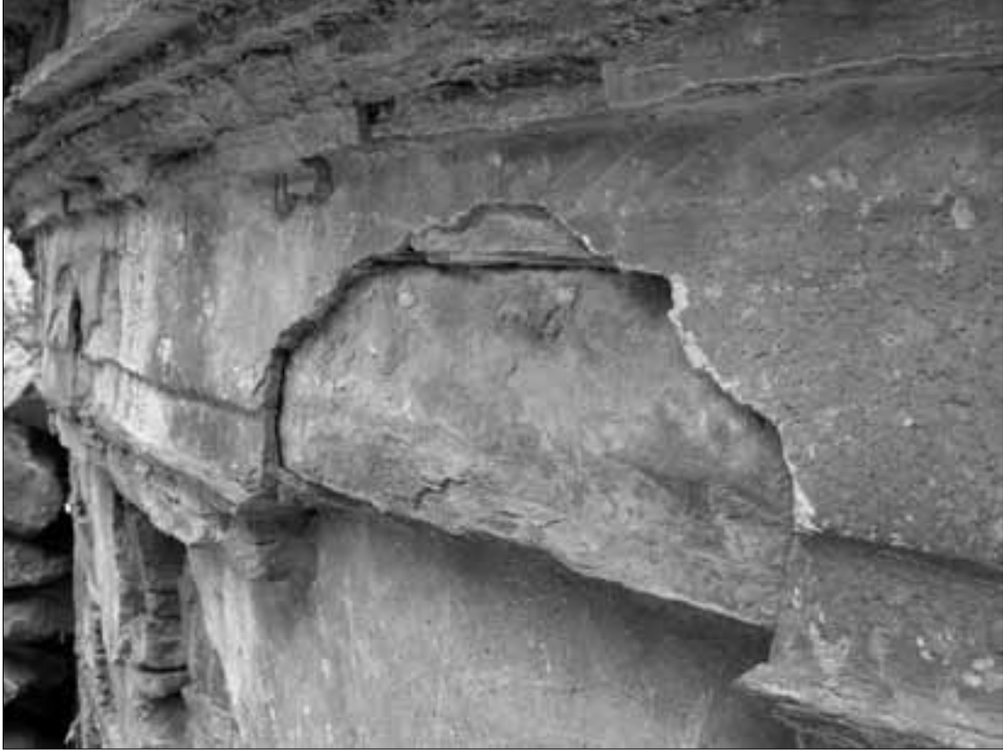
Fig. 301. Abbasahebchina. Stupa C. SE side, 3 rd storey; modillions of pilasters, stretch of architraved and bracketed cornice; plaster remains. (Spagnesi 2005).
