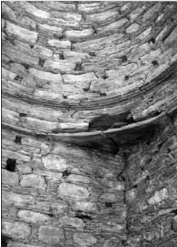
Fig. 447. Abbasahebchina, vihara F. Inside the aedicula (B); dome springer lying on slabs; detail of SW side with corner slabs and overlying band (F, G). (Taddei 1957; Neg. CS).
