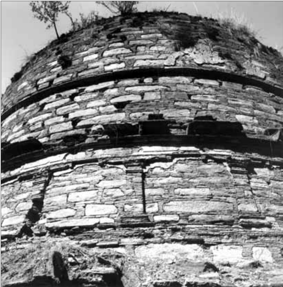
Fig. 240. Abbasahebchina. Stupa A. Lato SE side, 3 rd storey (drum), 4 th storey (transition storey of the composite dome), 5 th storey (raised dome); with remains of plaster. (Kuwayama 1993).
