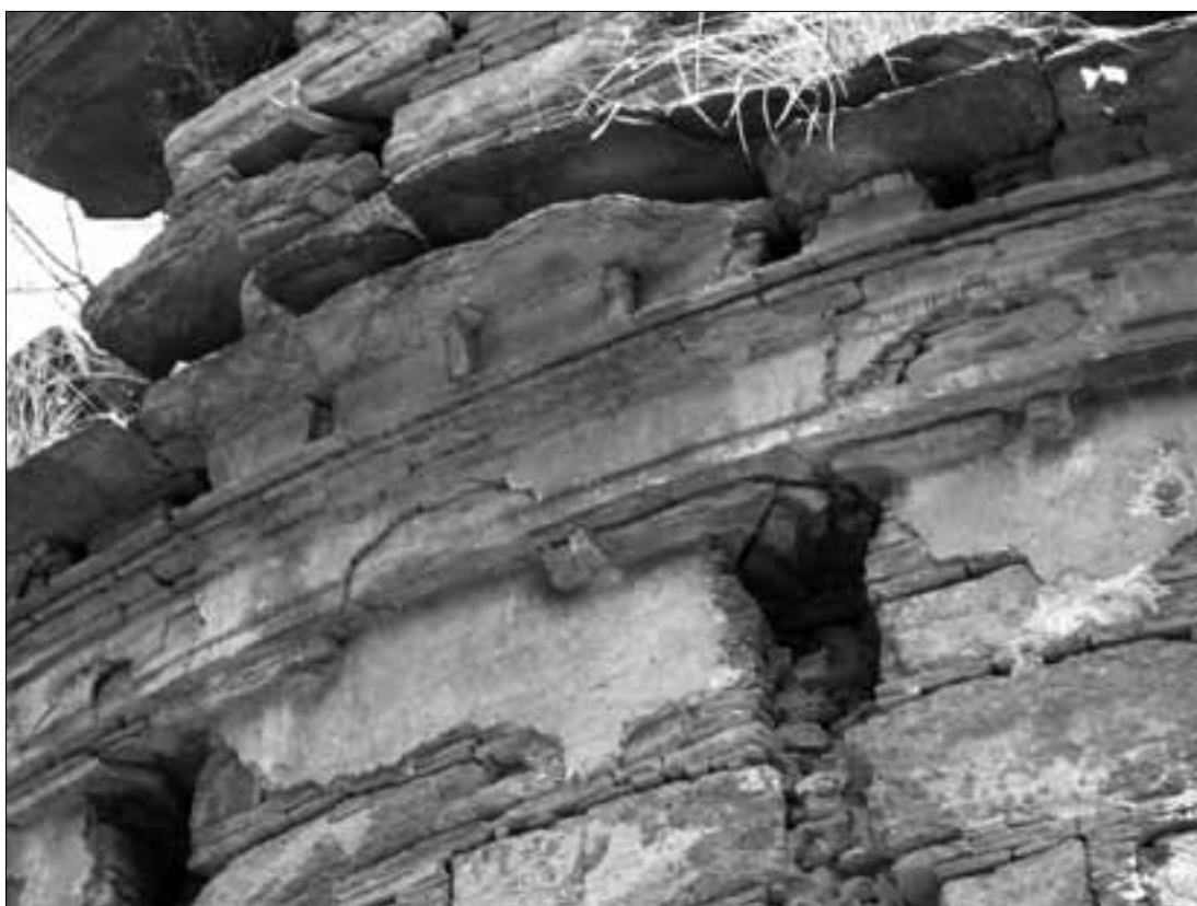
Fig. 300. Abbasahebchina. Stupa C. SE side, 3 rd storey; modillions of pilasters, stretch of architraved and bracketed cornice; plaster remains. Detail. (Spagnesi 2005).
