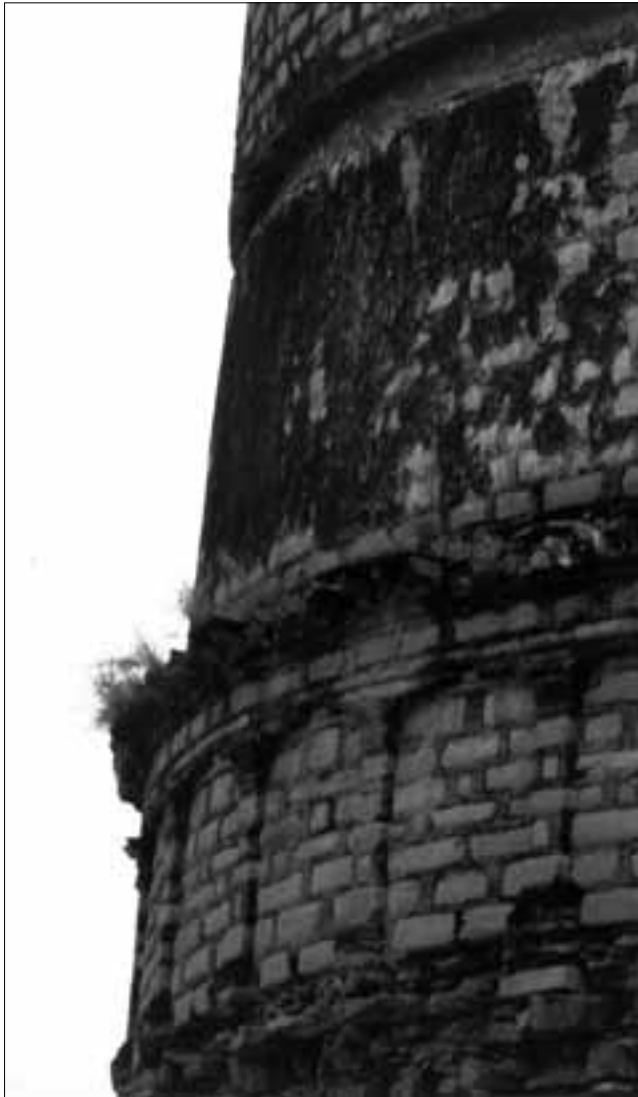
Fig. 143. Stupa of Shankardar. NW side; 3 rd storey (drum), 4 th and 5 th storey: composite dome with transition storey, recess for projecting small slabs, and dome springer. (Sabelli 1993).
