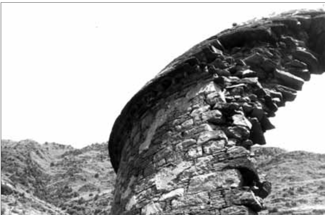
Fig. 521. Gumbatuna, Vihara. SW side; upper part of the outer wall of the cell showing remains of plaster, cornice and the beginning of the dome. (Faccenna 1960; Neg. CS).
