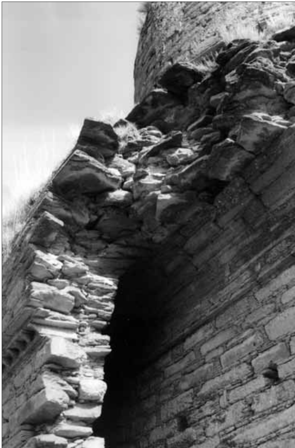
Fig. 473. Vihara of Gumbat. E side; S corridor, initial stretch of the vault springer. (Spagnesi 2004).
