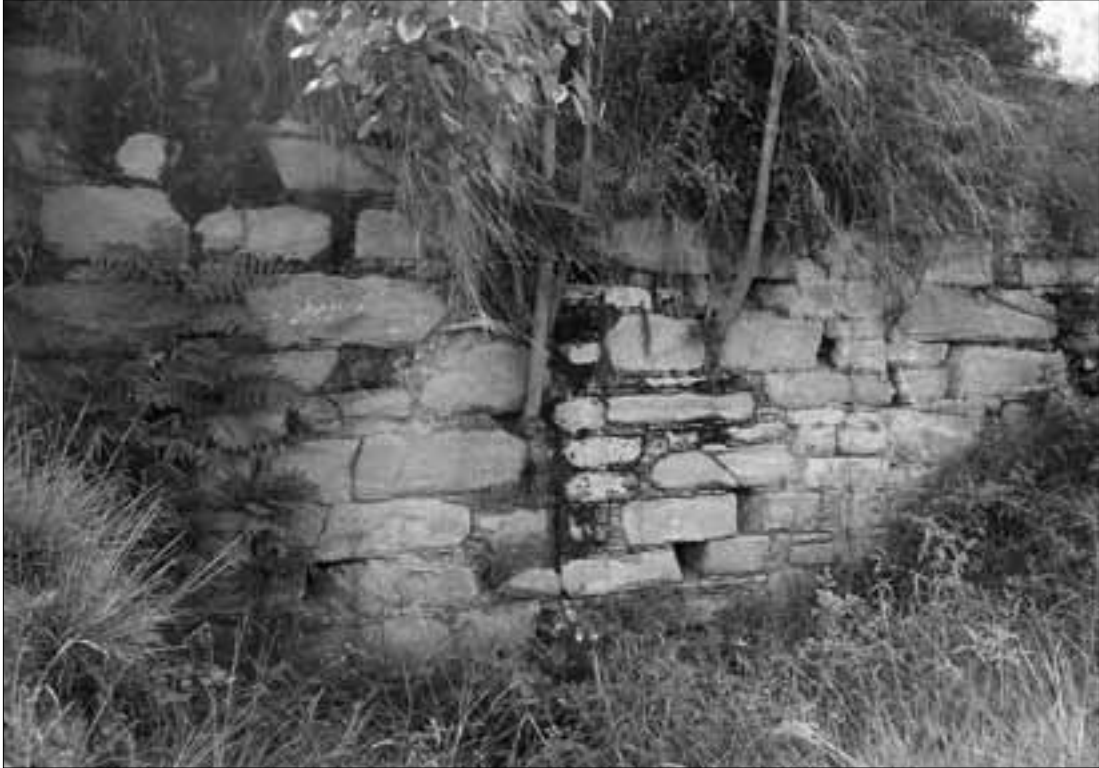
Fig. 30. Stupa of Jurjurai. 1 st storey, detail of a corner with pilaster. (Spagnesi 2005).
